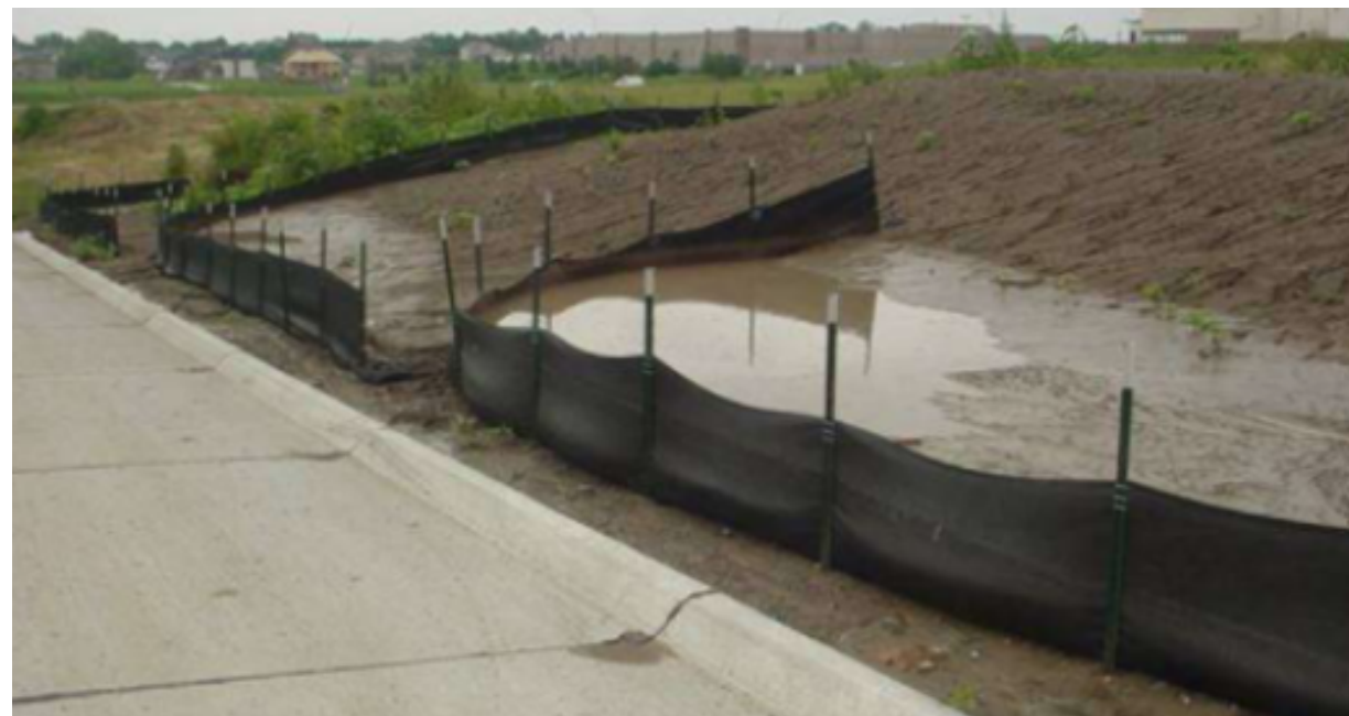
Figure 6-3. Typical Example of a Silt Trap fence
