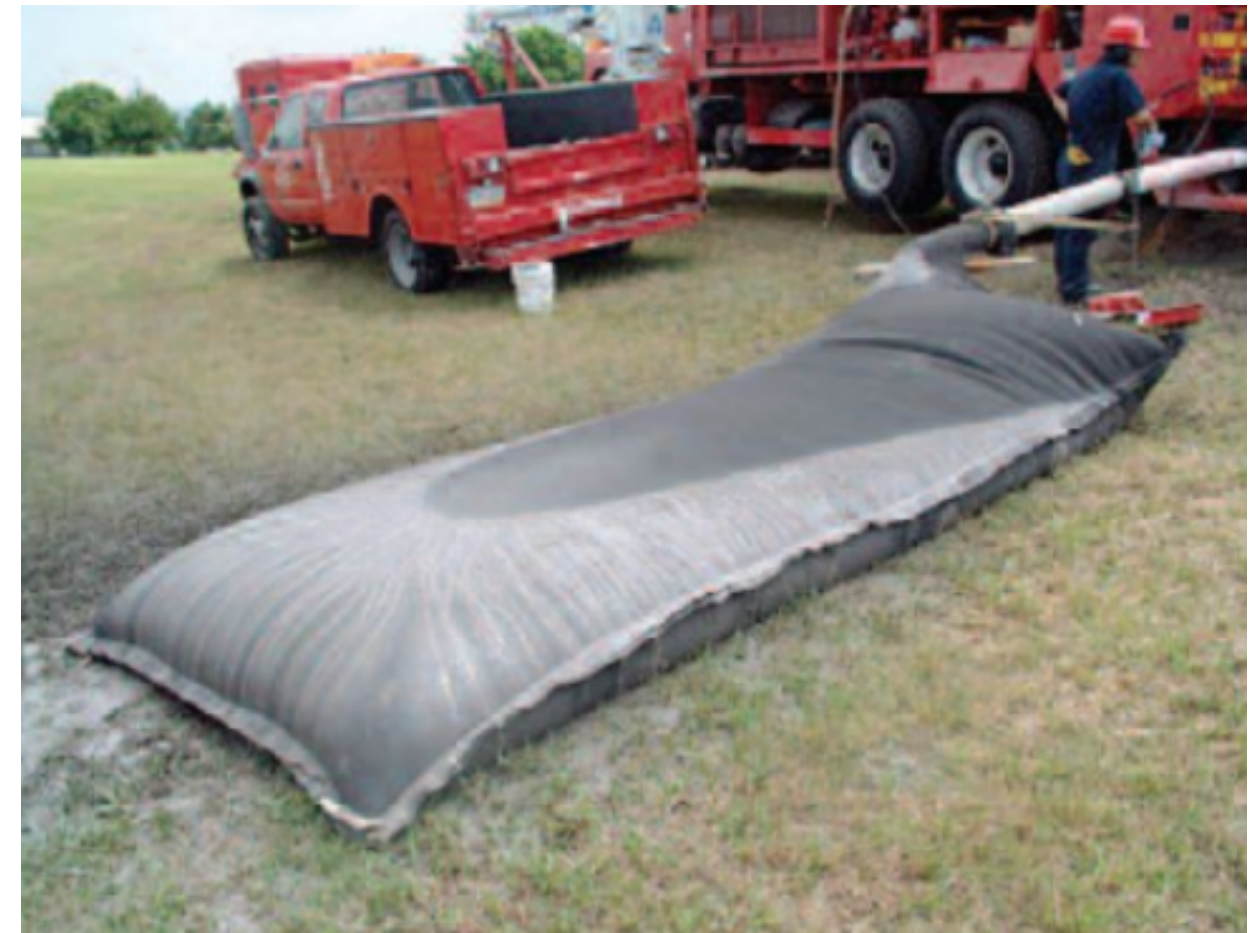
Figure 6-2. Typical Example of Settlement Tanks
